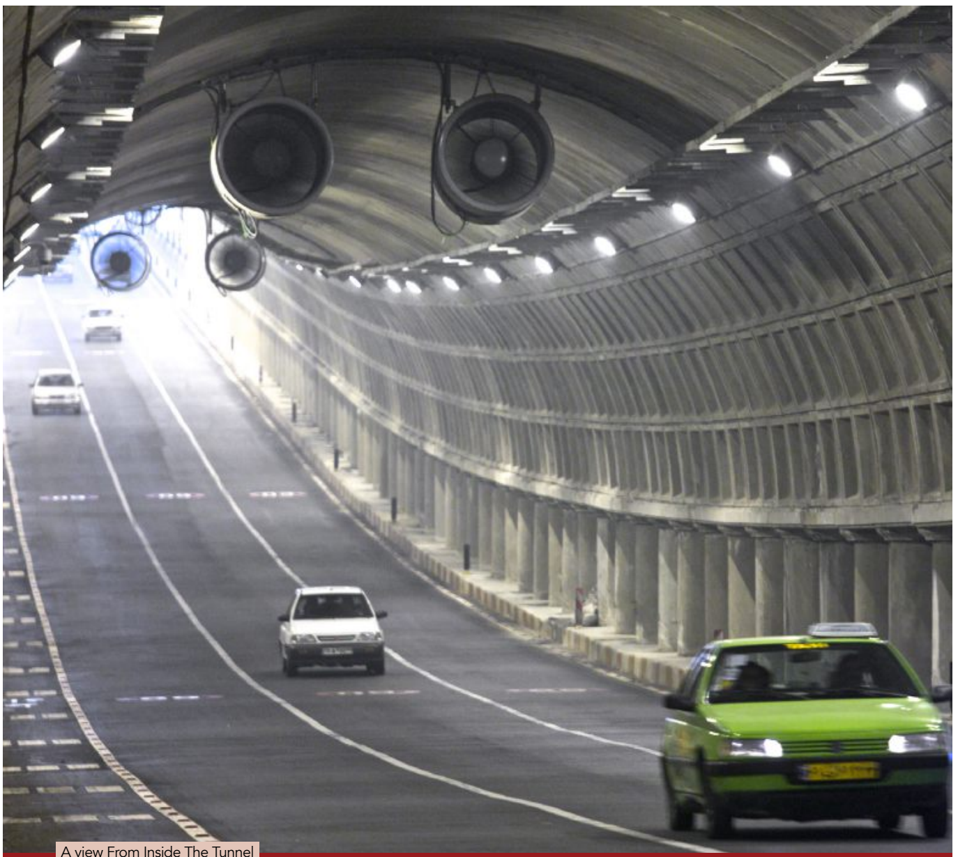
A view From Inside The Tunnel
