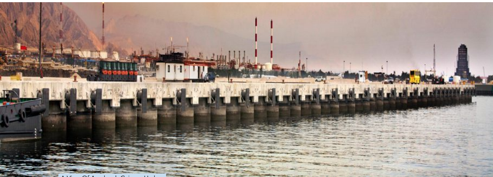
A View Of Assaluyeh Caisson Harbor
