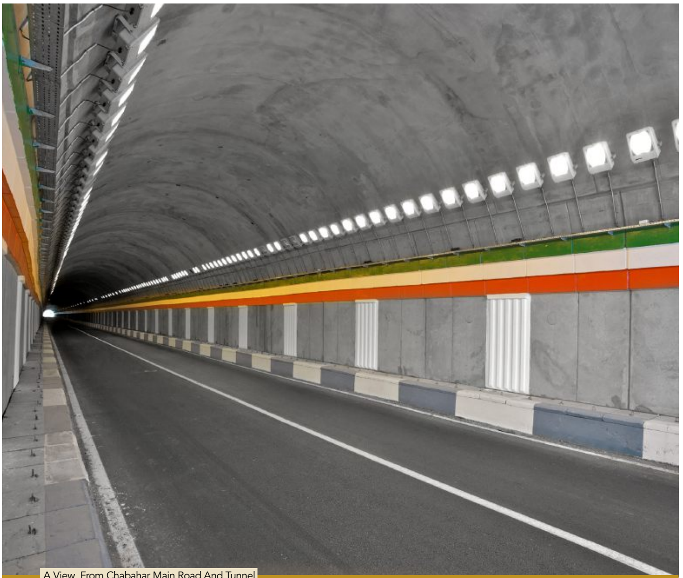
A View From Chabahar Main Road And Tunnel
