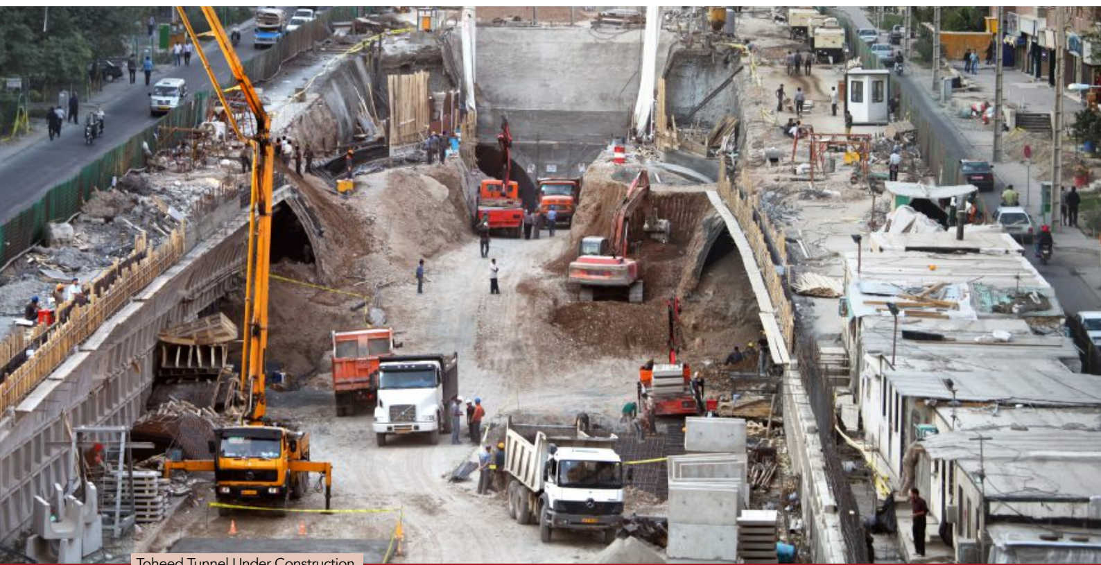
Toheed Tunnel Under Construction
