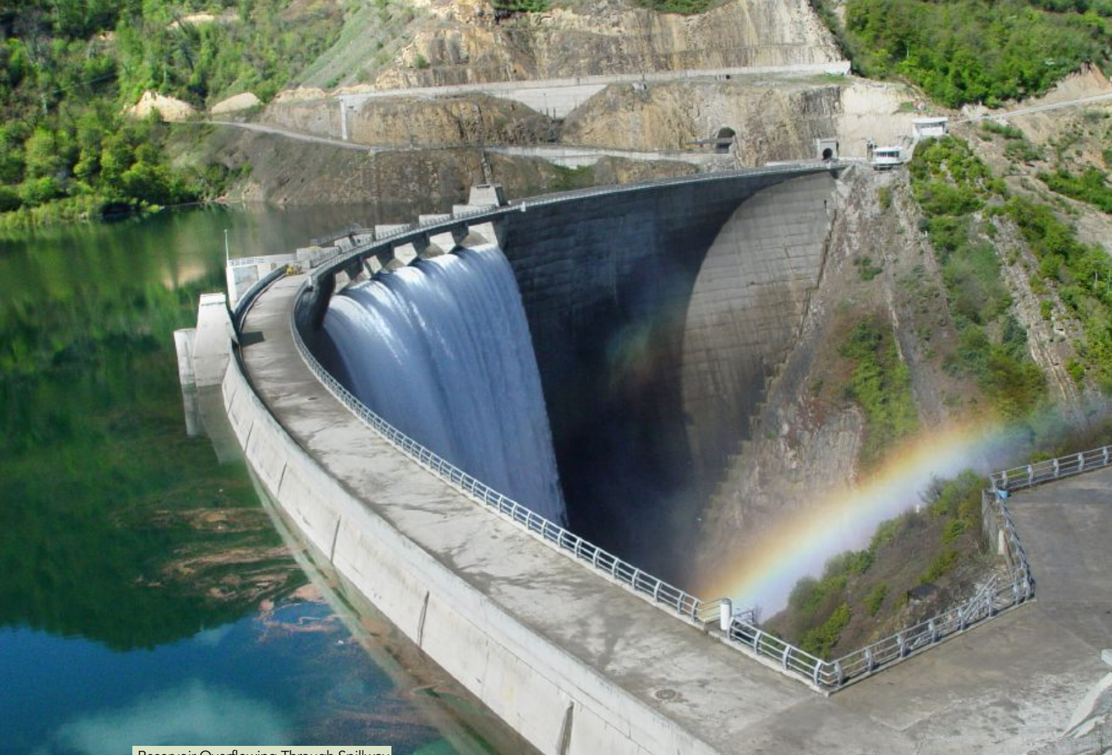
Reservoir Overflowing Through Spillway
