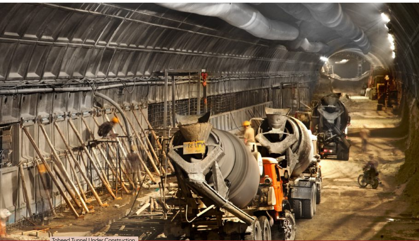
Toheed Tunnel Under Construction
