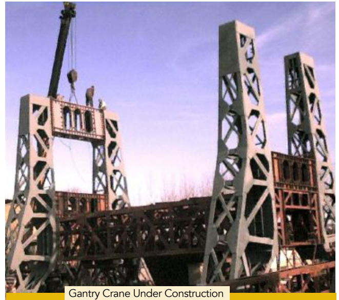
Gantry Crane Under Construction
