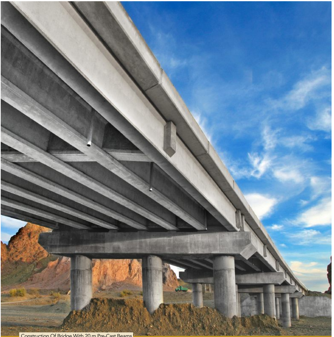
Construction Of Bridge With 20 m Pre-Cast Beams
