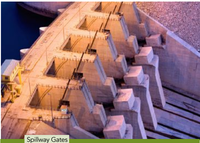
Spillway Gates
