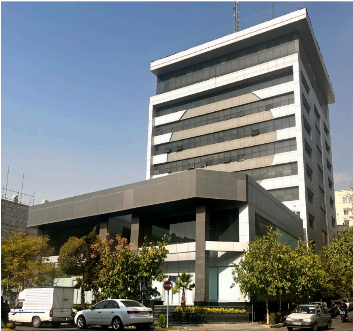
Perlite Borgeh Construction Consortium Main Office
