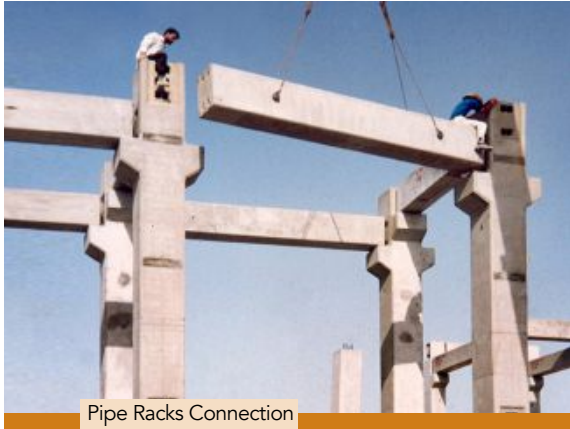
Pipe Racks Connection
