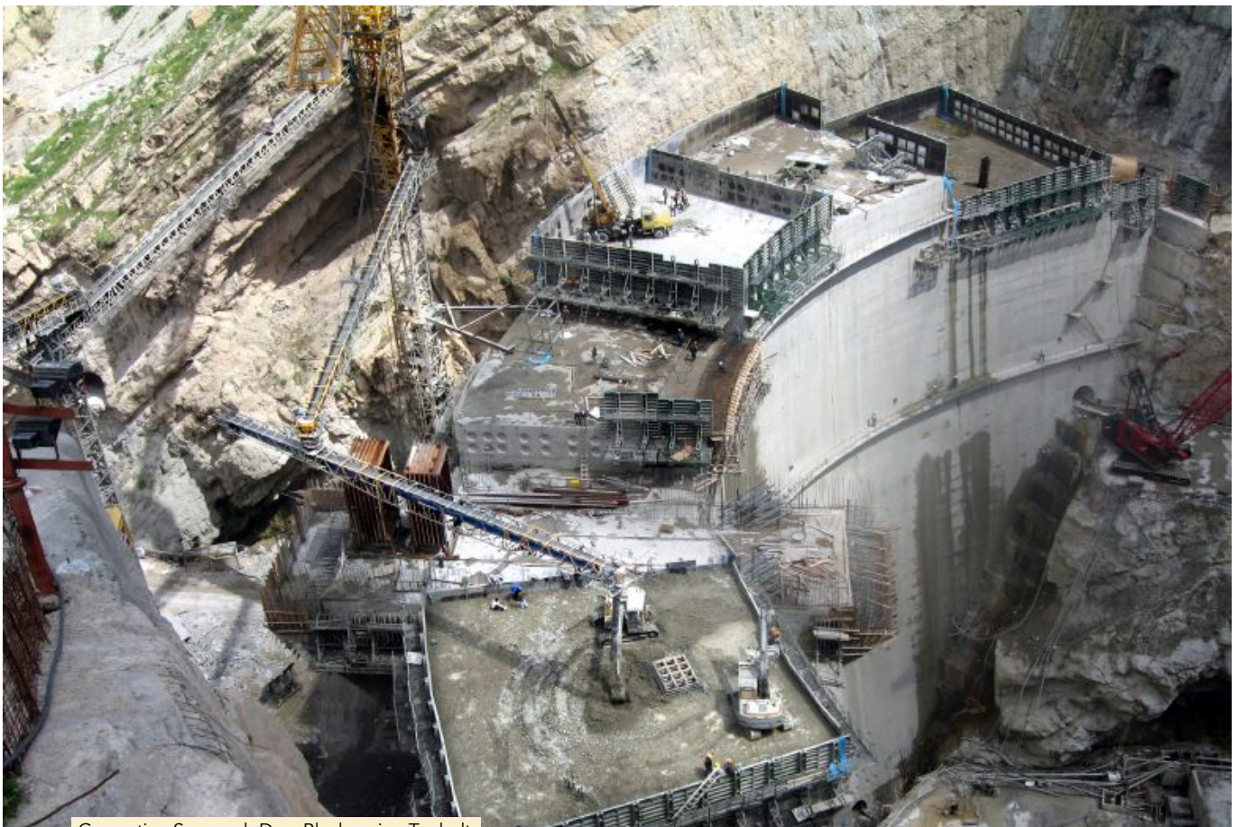
Concreting Seymareh Dam Blocks using Topbelt
