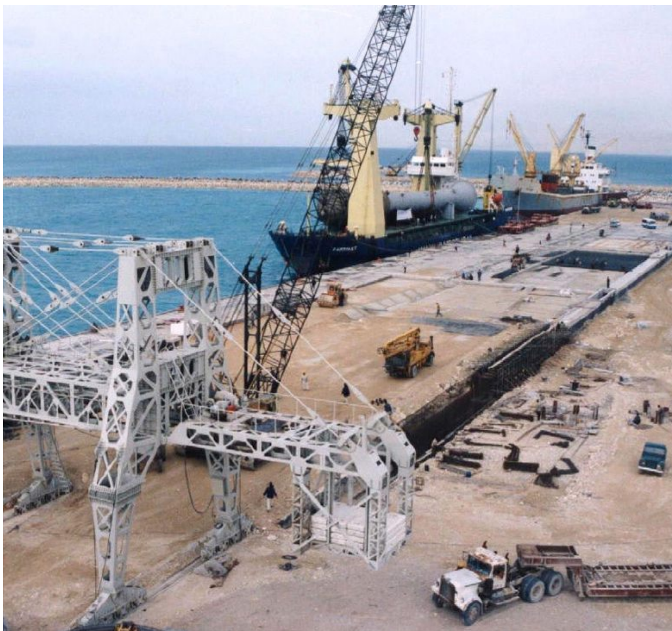
Harbor Ready For Operation
