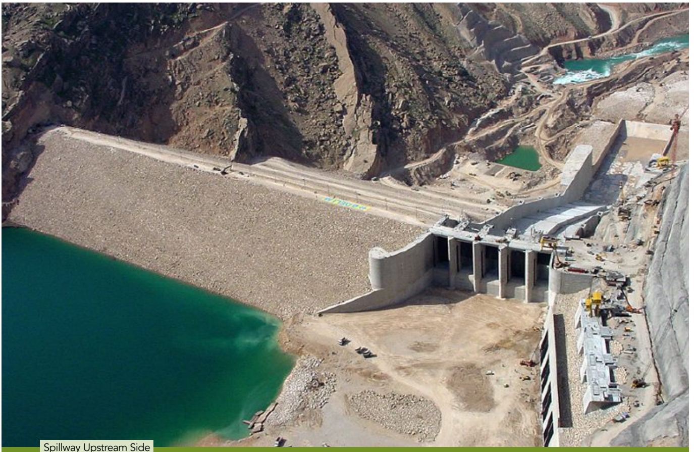
Spillway Gates
