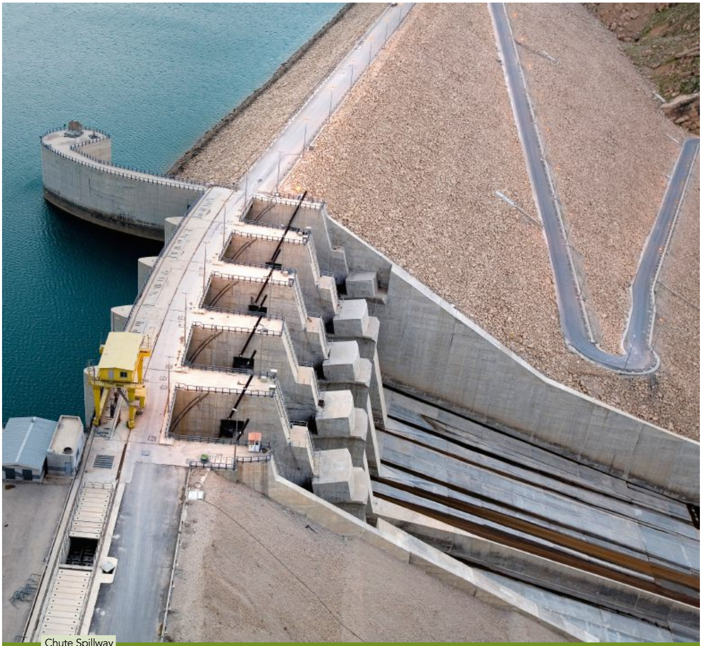
Chute Spillway
