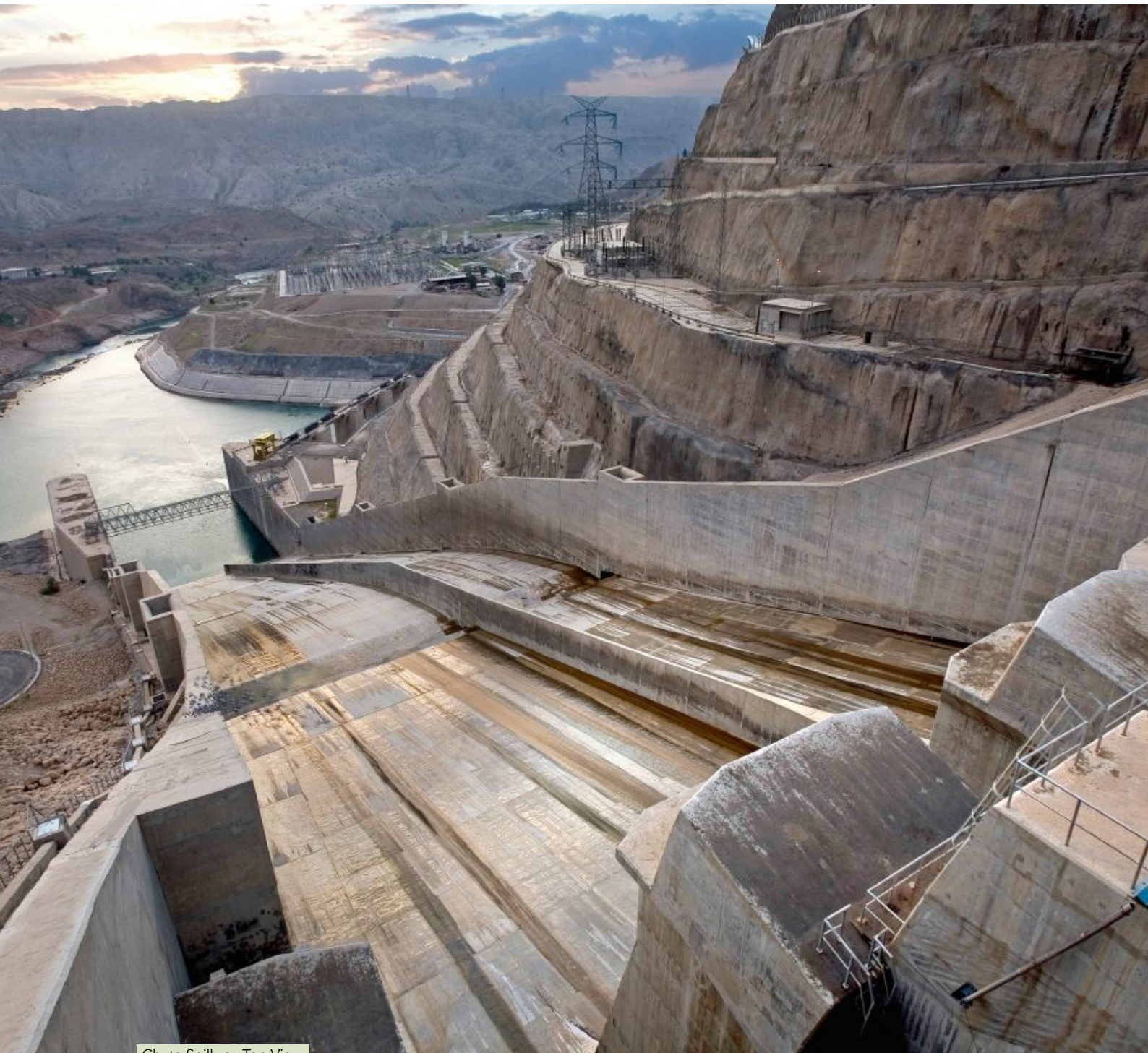
Chute Spillway Top View
