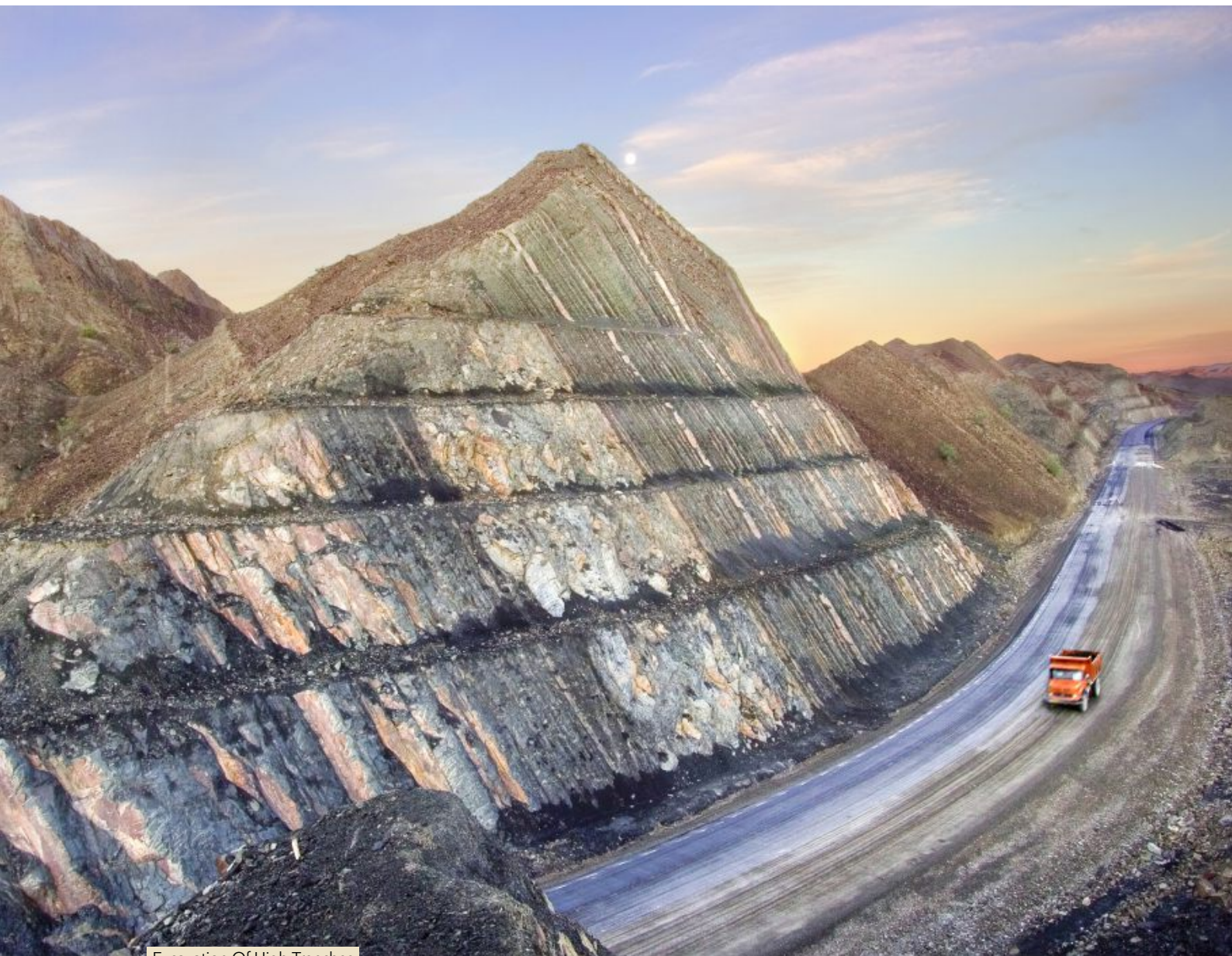
Excavation Of High Trenches
