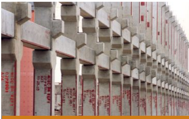
High Elevation Pipe Racks
