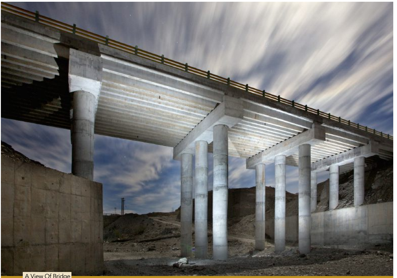
A View Of Bridge
