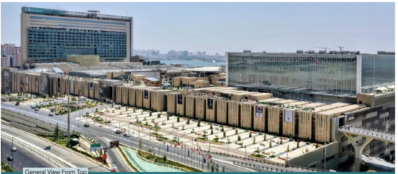
General View From Top
