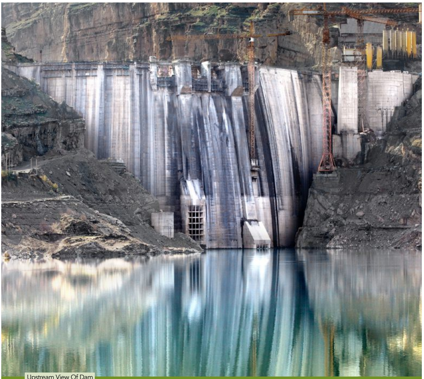
Upstream View Of Dam
