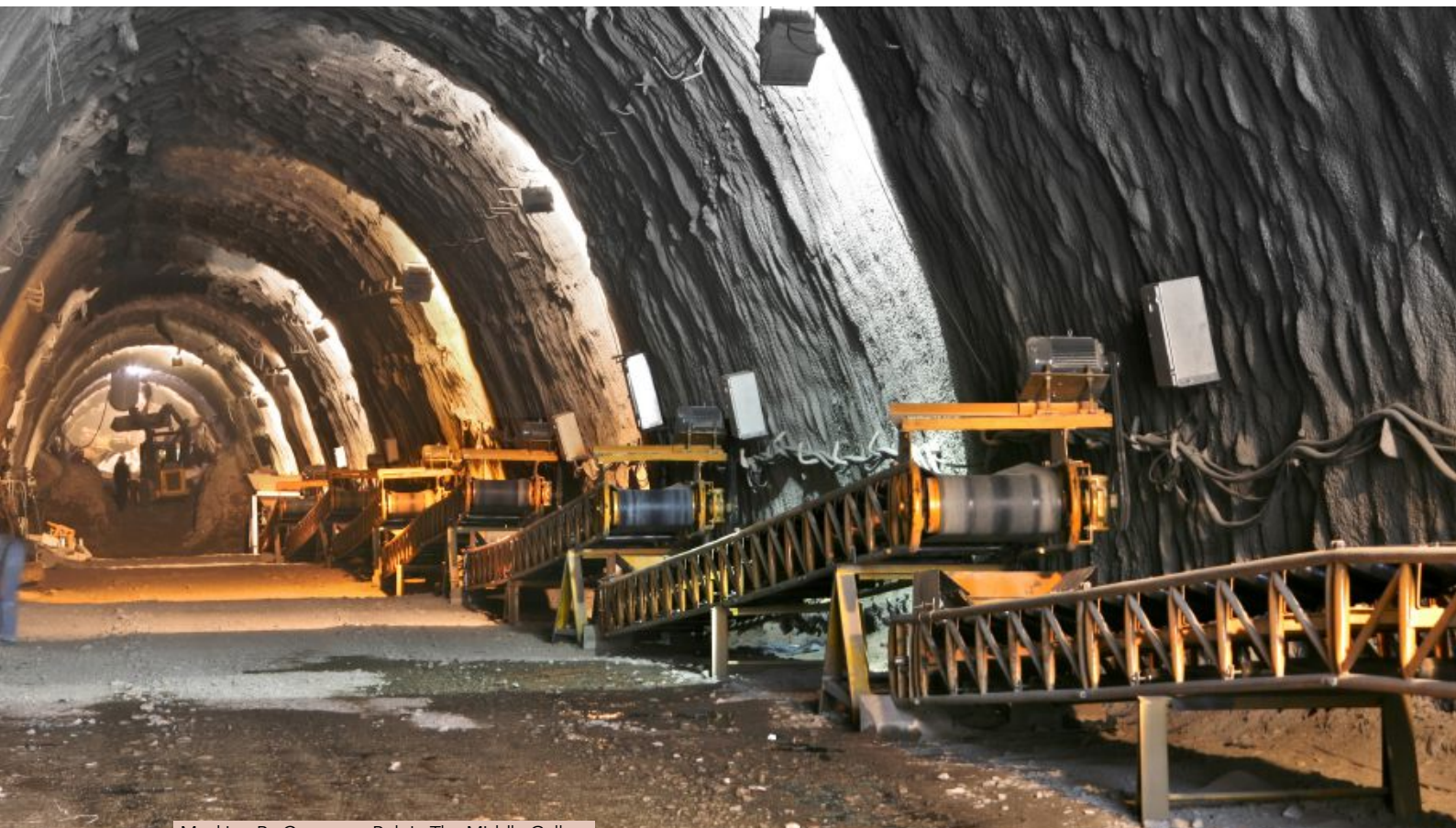
Mucking By Conveyor Belt In The Middle Gallery
