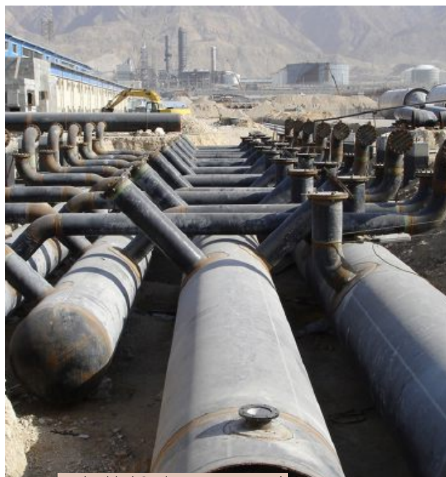
Embedded Cooling Water Network
