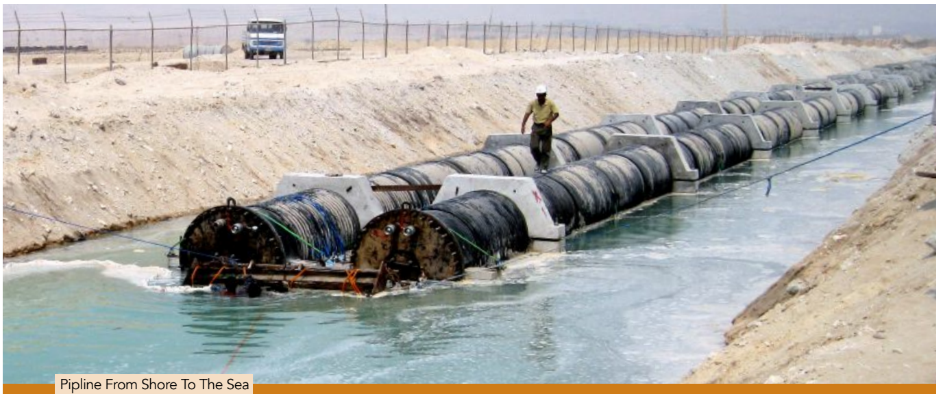
Polyethylene Pipeline Connection
