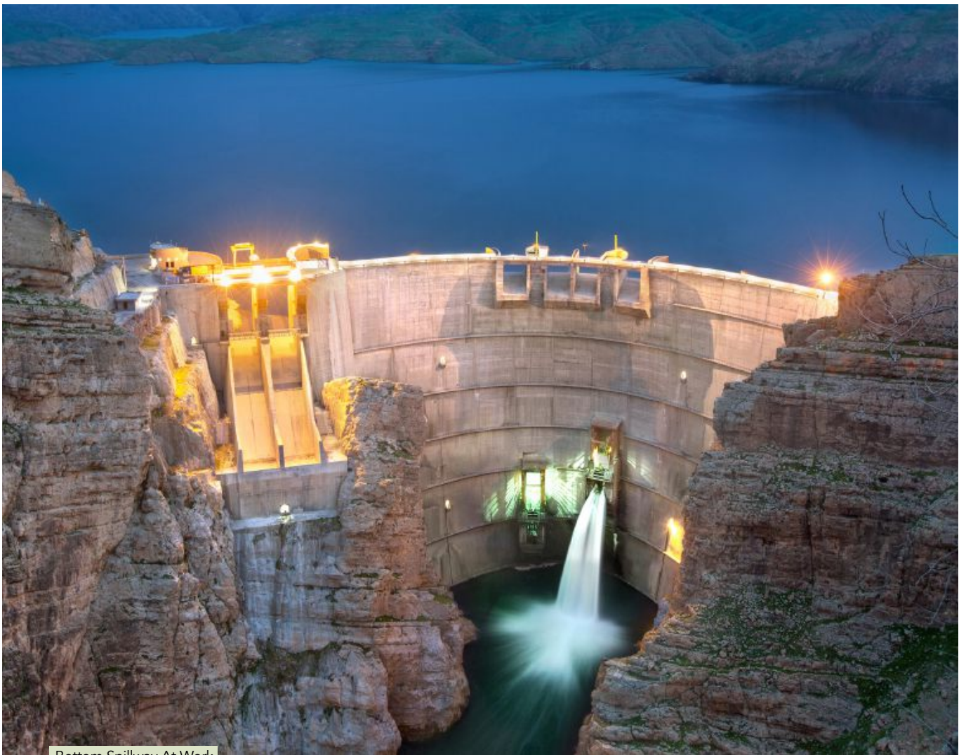
Bottom Spillway At Work
