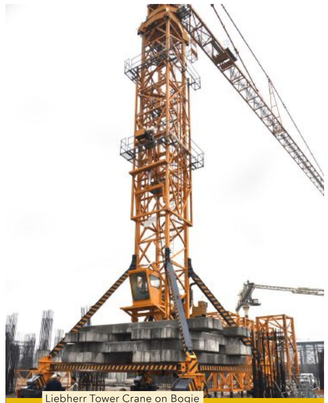
Liebherr Tower Crane on Bogie
