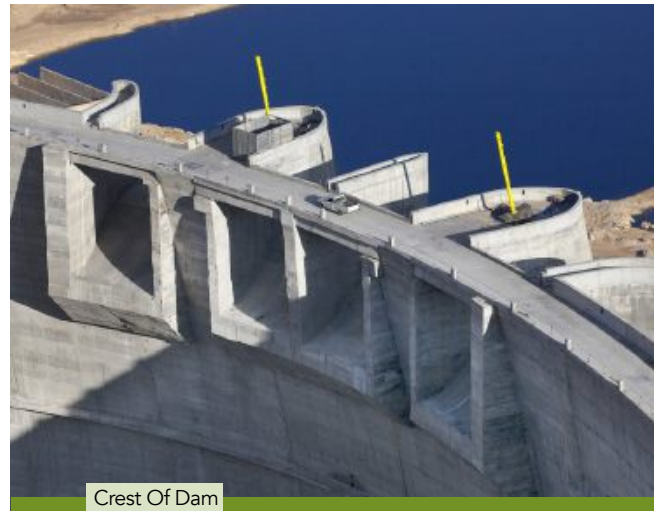
Crest Of Dam
