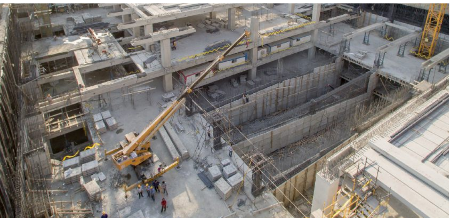
Installation of 18m beam using two cranes
