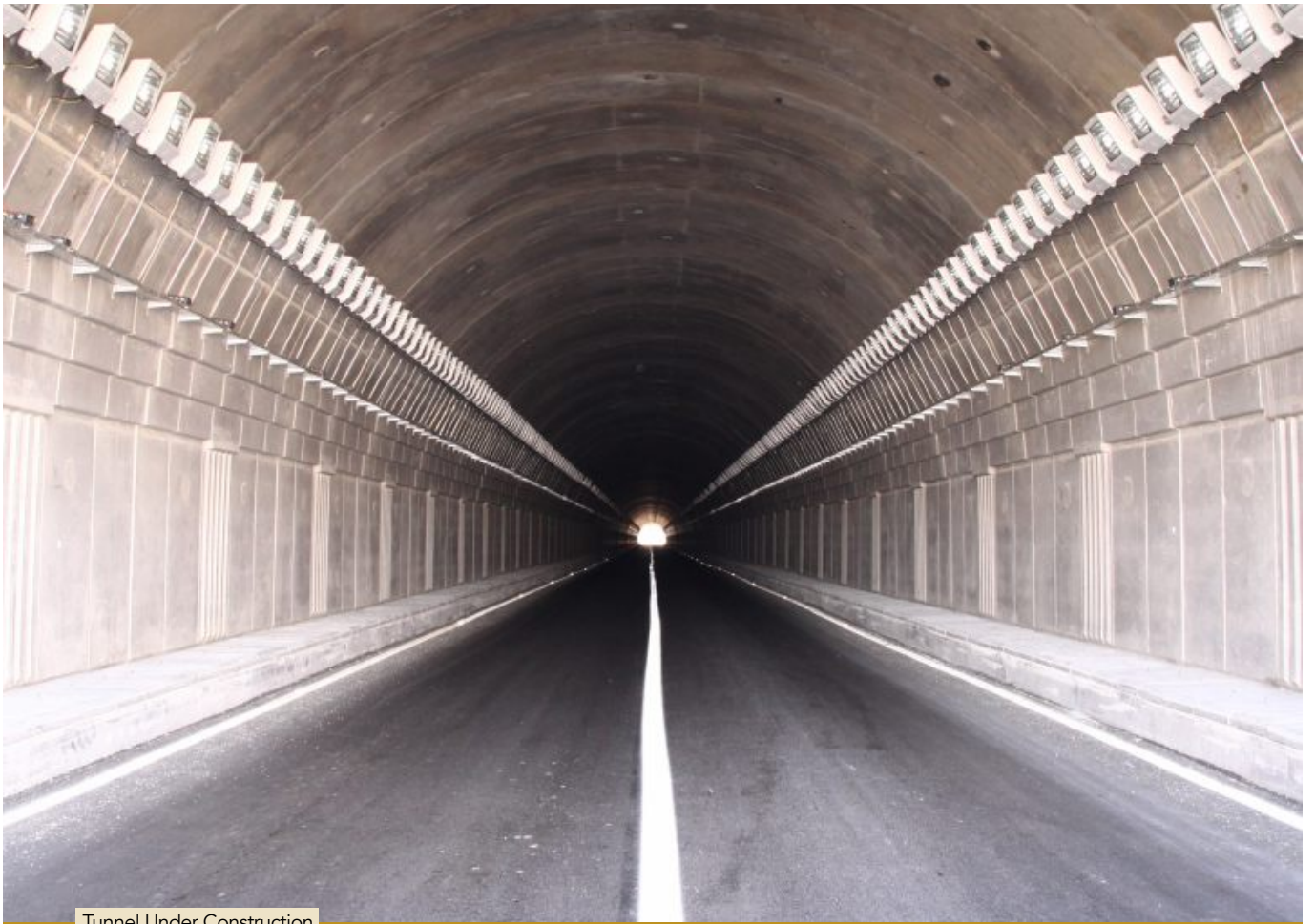
Tunnel Under Construction
