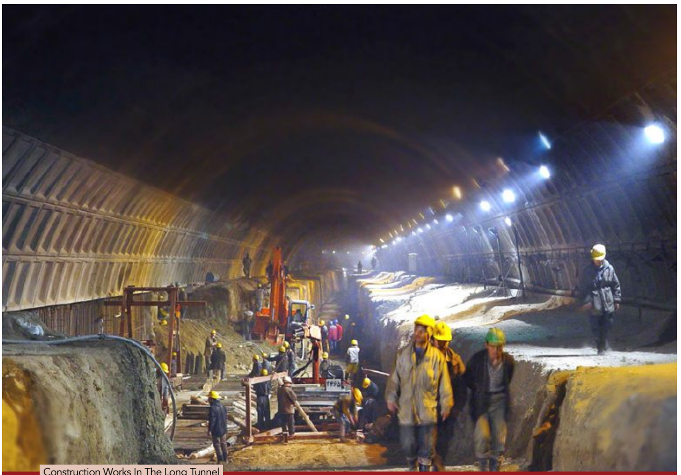
Construction Works In The Long Tunnel
